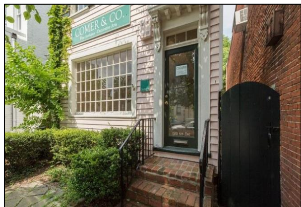
An example of ground floor commercial conversion
