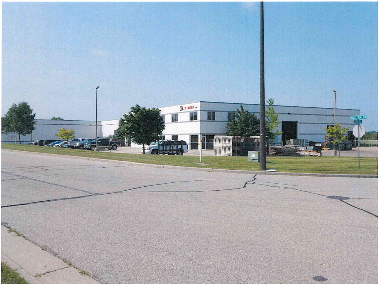
NORTHEAST CORNER LOOKING SOUTHWEST AT EXISTING ENTRY
