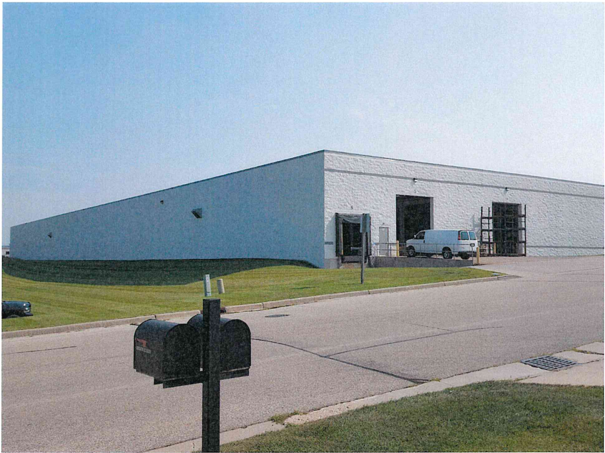
SOUTHWEST CORNER LOOKING NORTHEAST
