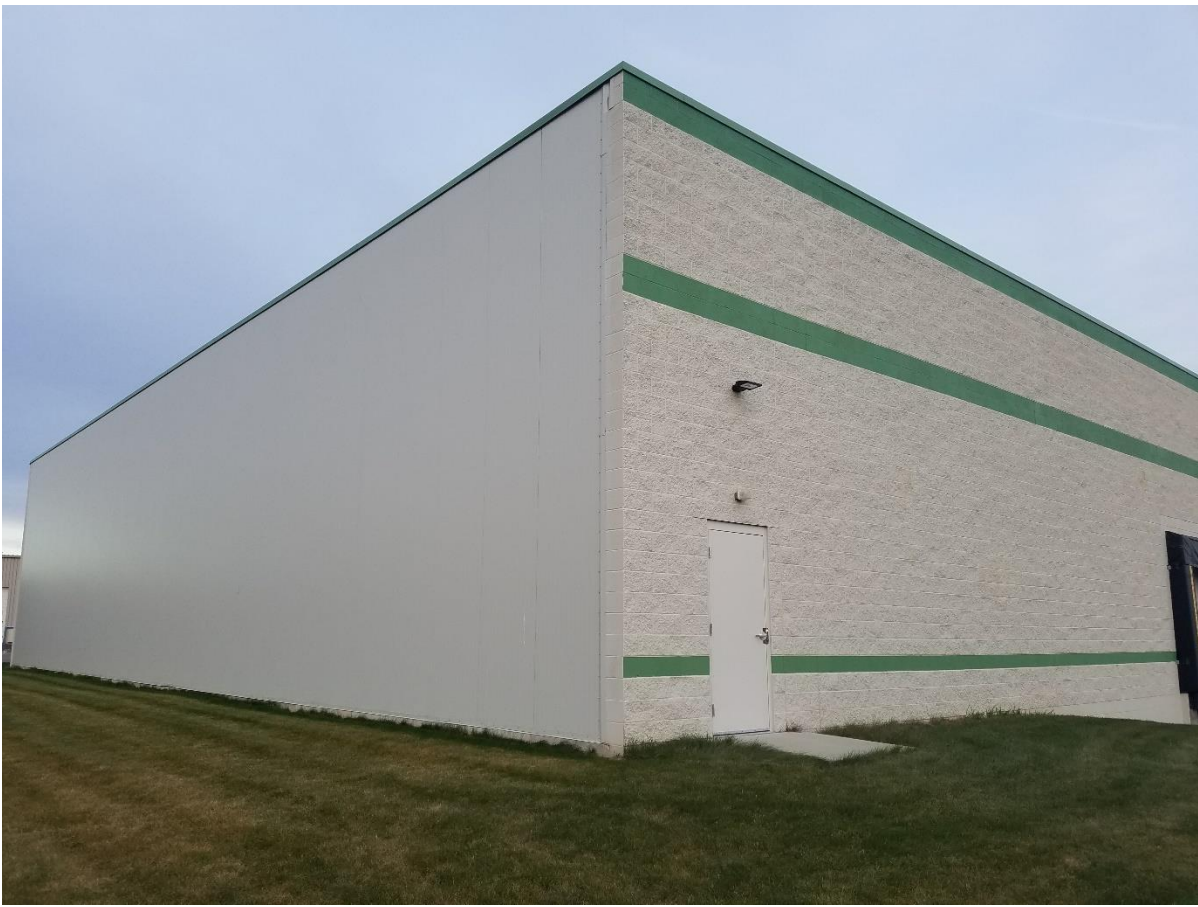
CLOSE-UP CORNER VIEW OF EXISTING MASONRY AND METAL PANEL MATERIALS TO BE MATCHED
