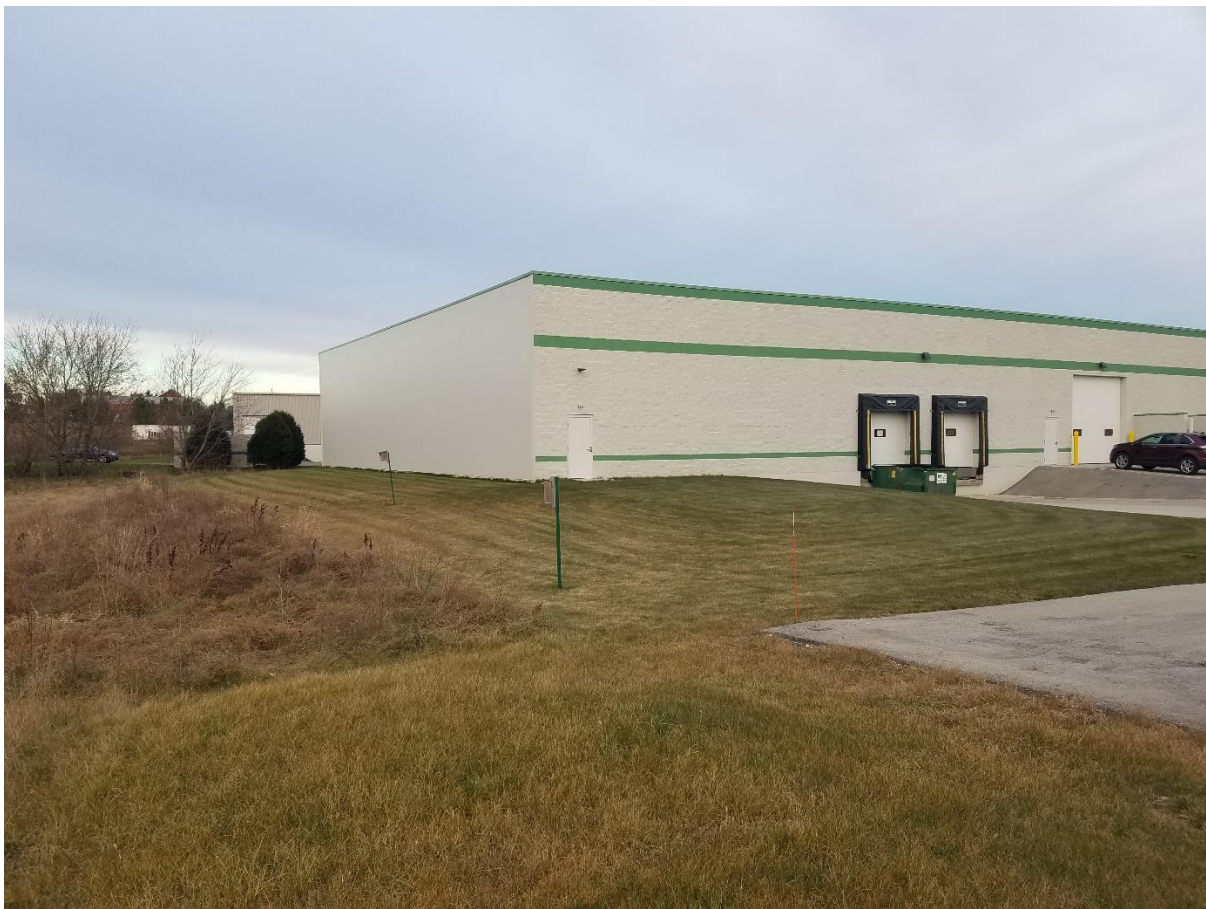
SOUTHWEST CORNER LOOKING NORTH TOWARD LOCATION OF PROPOSED ADDITION
