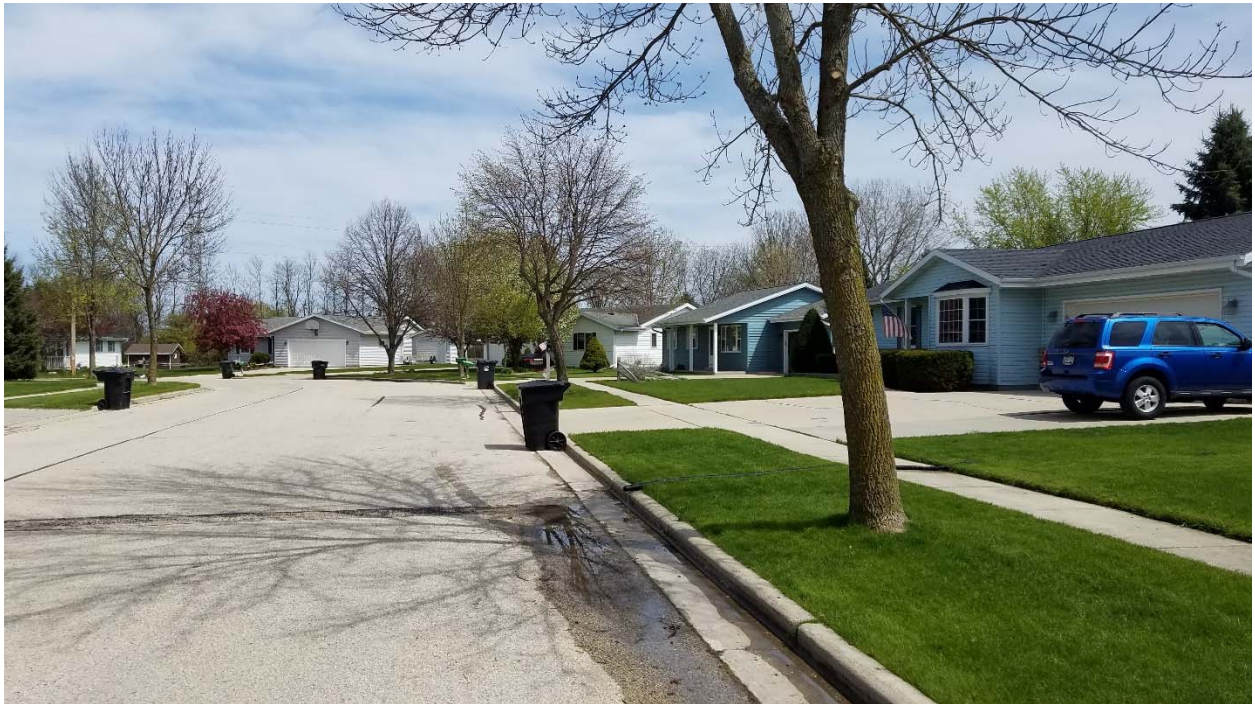
Sump pump discharge from W194 N16013
