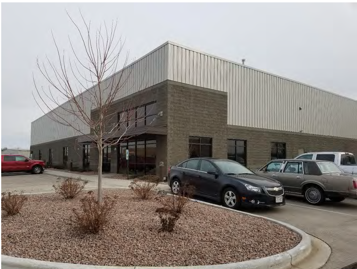
NORTHWEST CORNER LOOKING SOUTHEAST AT EXISTING MAIN ENTRANCE
