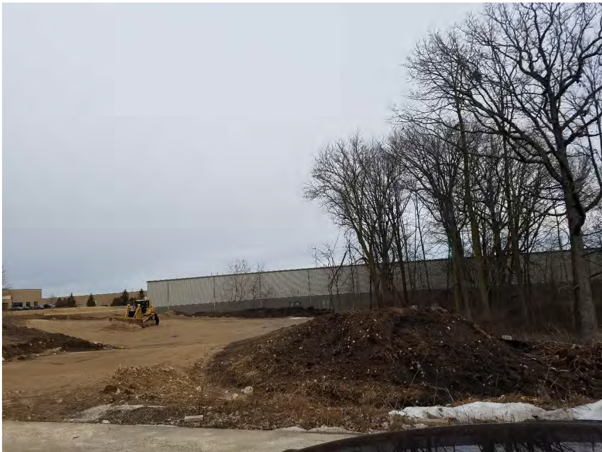
LOOKING EAST TOWARD PROPOSED ADDITION WITH WETLANDS TO THE SOUTH
