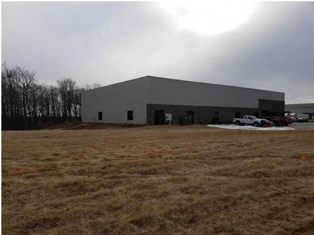
NORTHEAST CORNER LOOKING SOUTHWEST TOWARD EXISTING BUILDING
