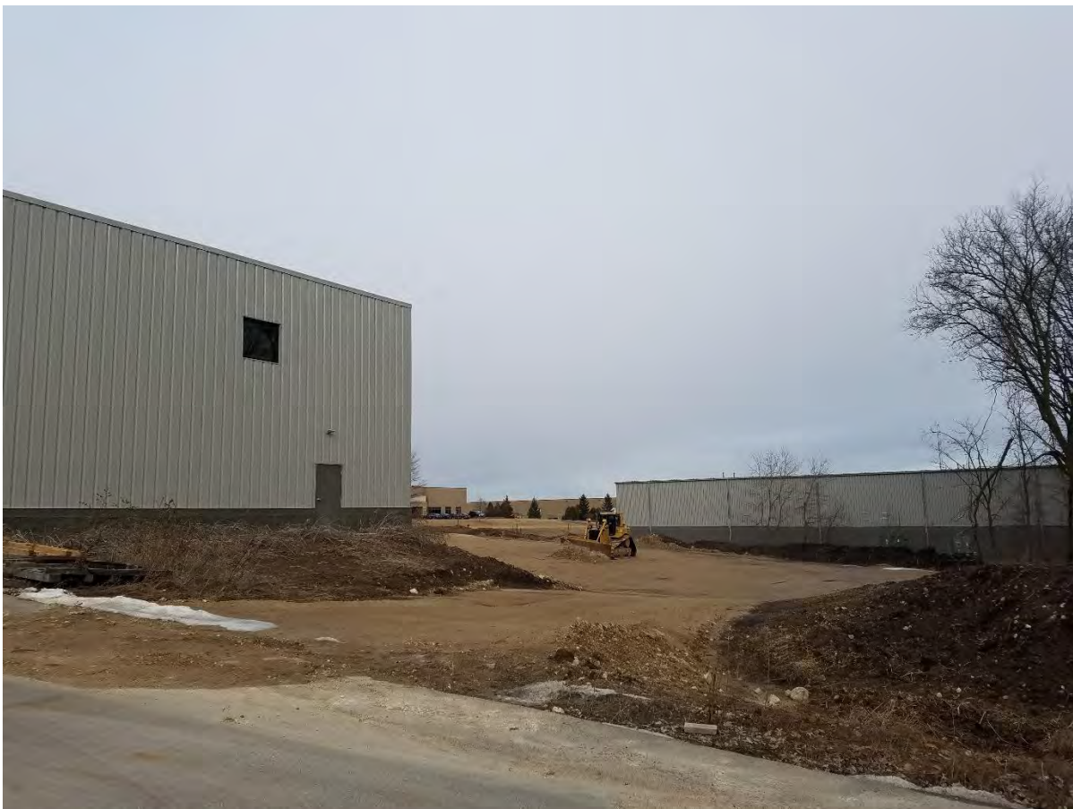
VIEW OF SOUTH SIDE OF EXISTING BUILDING AT LOCATION OF PROPOSED ADDITION
