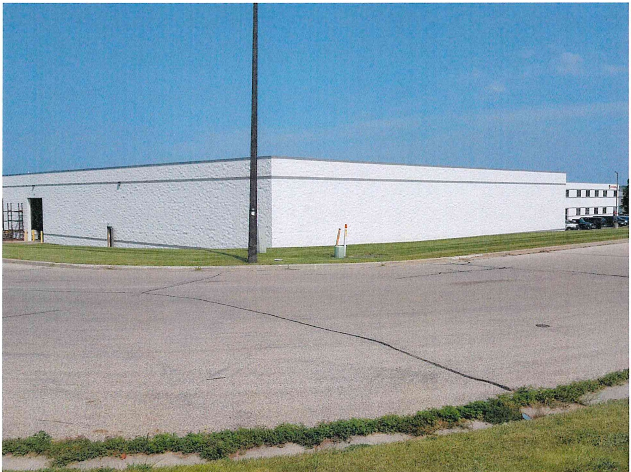
SOUTHEAST CORNER LOOKING NORTHWEST
