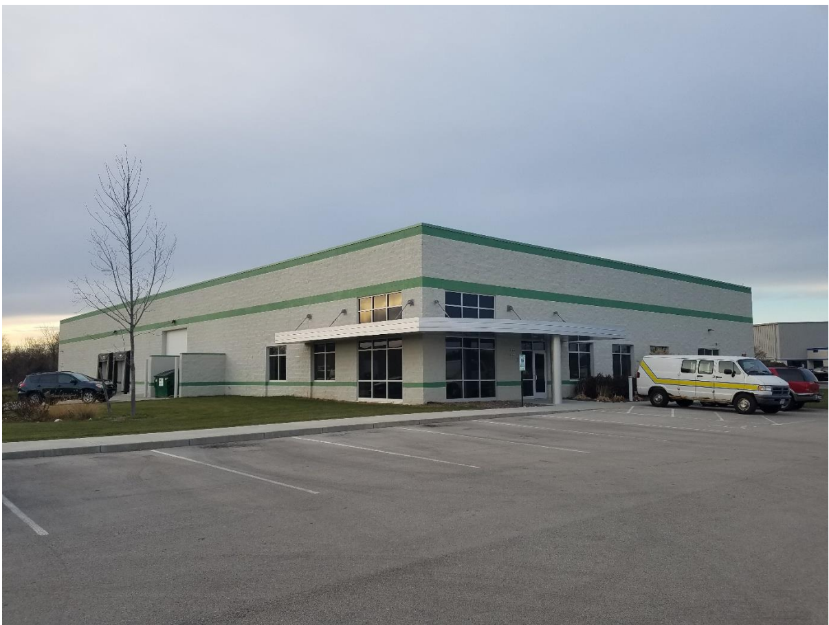
SOUTHEAST CORNER LOOKING NORTHWEST AT EXISTING MAIN ENTRANCE
