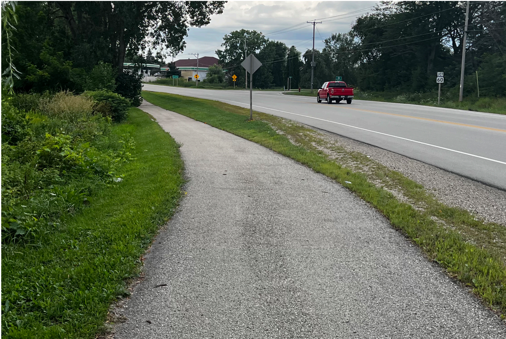
Existing Paved Multi-Use Path
