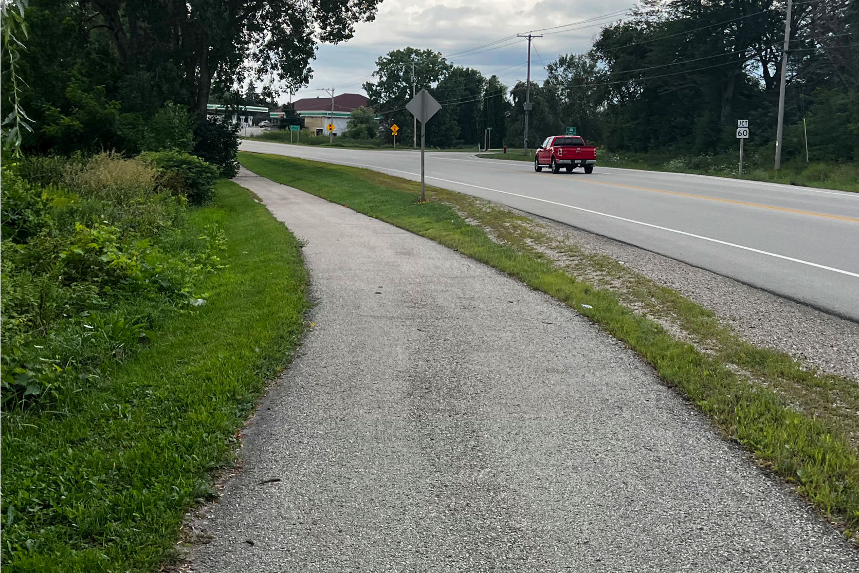
Existing Paved Multi-Use Path
