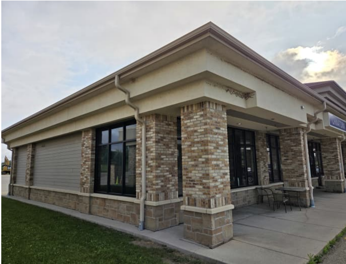
EXISTING RETAIL BUILDING
