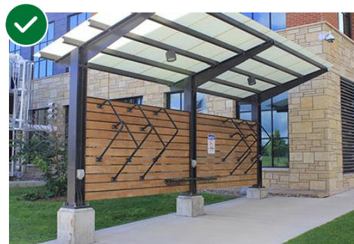
Exhibit 21-8. An example of a covered bicycle rack
