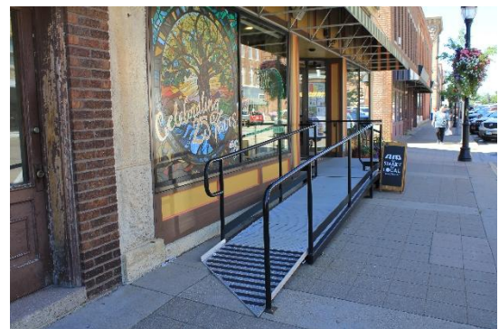
Exhibit 19-6. An example of an encroachment in a public sidewalk
