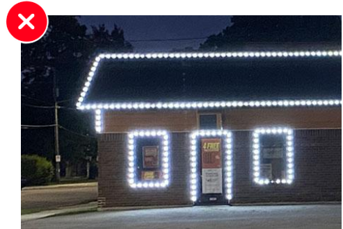
Exhibit 22-1. An example of prohibited lighting
