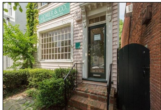
An example of ground floor commercial conversion
