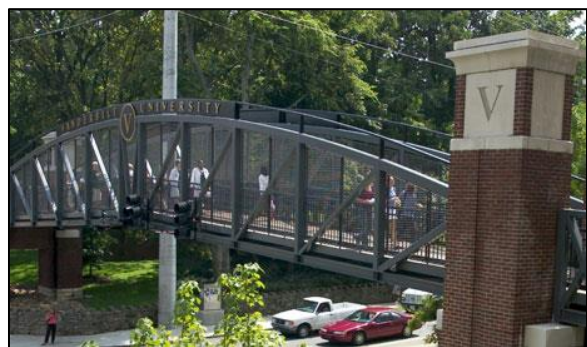
Bicycle and pedestrian bridges provide connections in areas with specific challenges and opportunities such as rail corridors and busy streets
