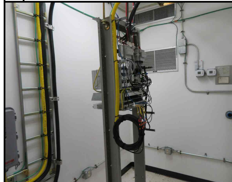
D EXISTING LTE RACK(S) TO BE REMOVED
