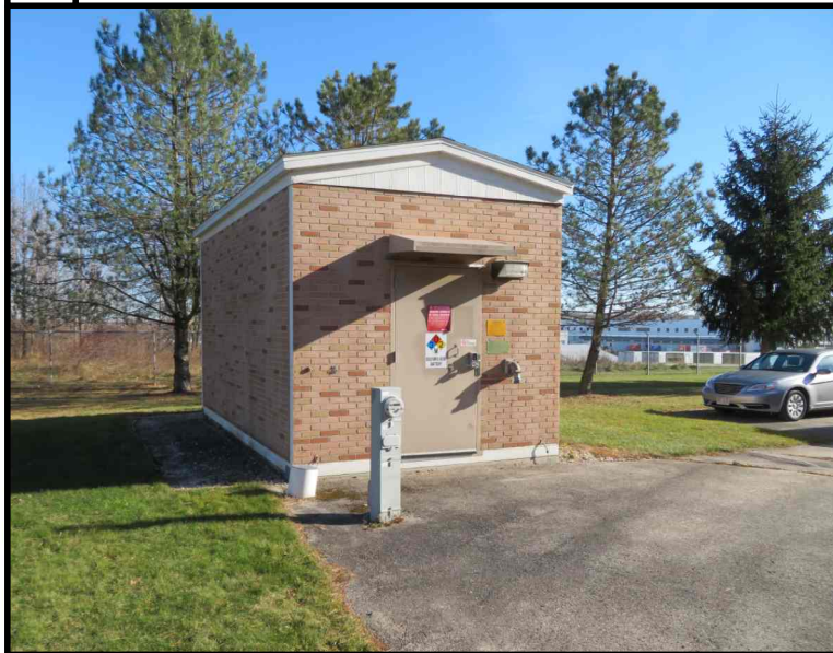
B COMPOUND OVERVIEW
