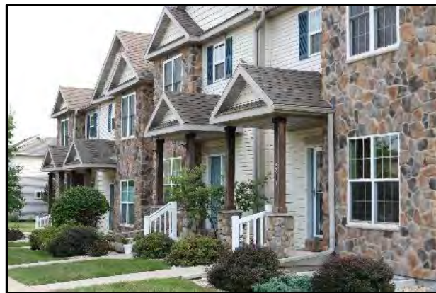
Figure 9 Sample image of a townhome building.
