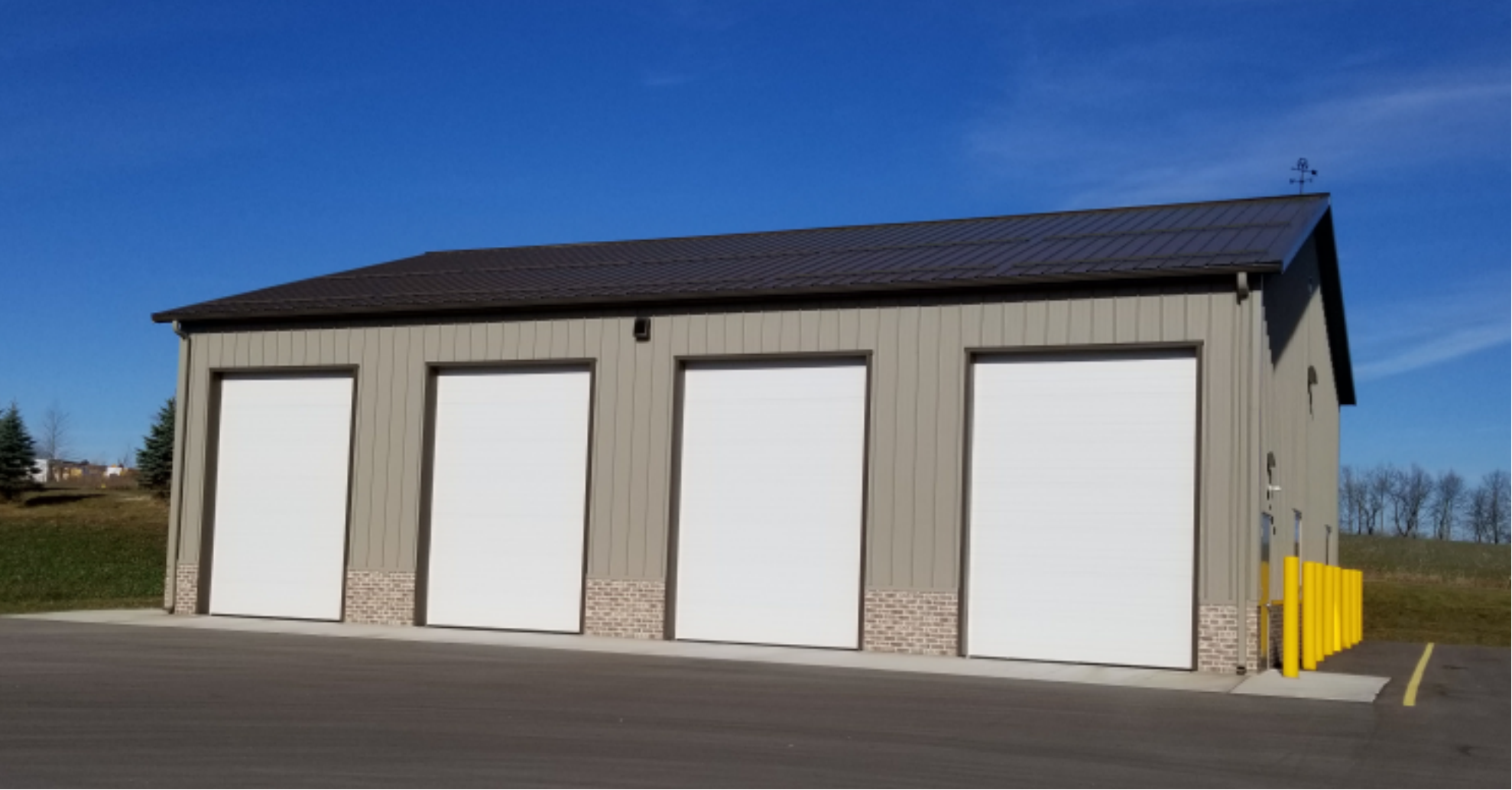
EXISTING BUILDING SOUTH FACADE
