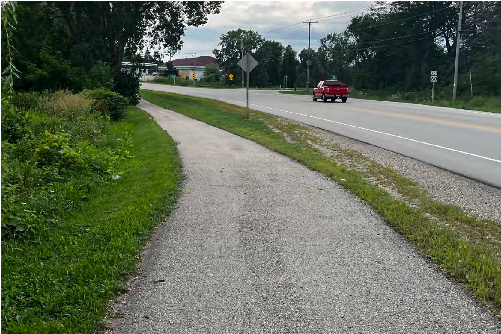
Existing Paved Multi-Use Path
