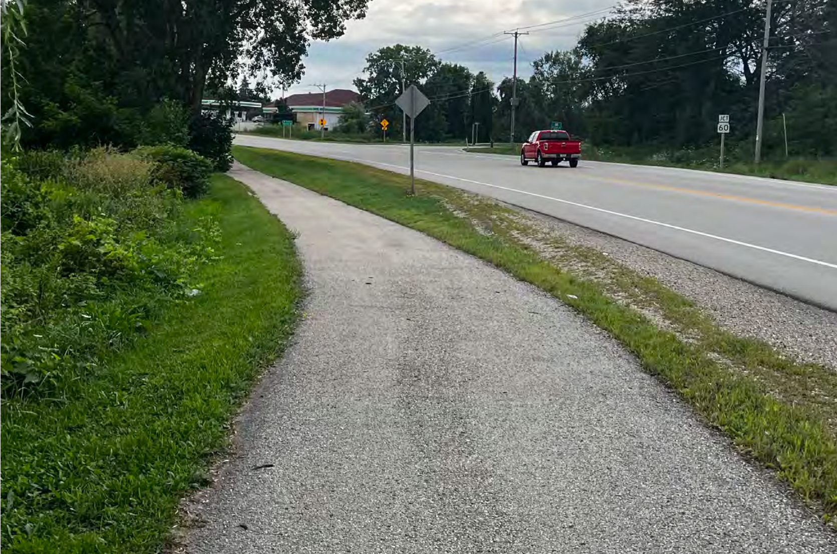
Existing Paved Multi-Use Path
