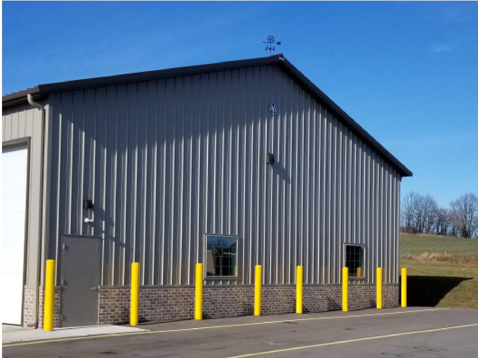
EXISTING BUILDING EAST FACADE
