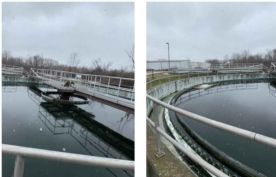
Final Clarifiers - Newer
