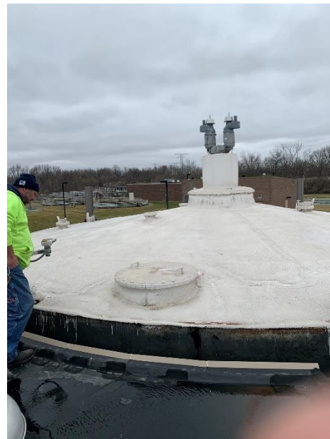
Digester Floating Truss and Gasholder Covers
