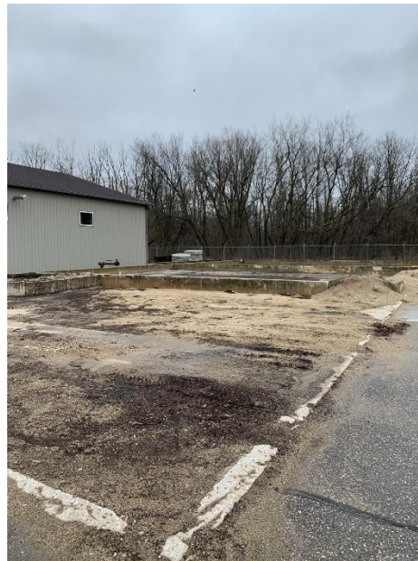
Sludge Drying Beds
