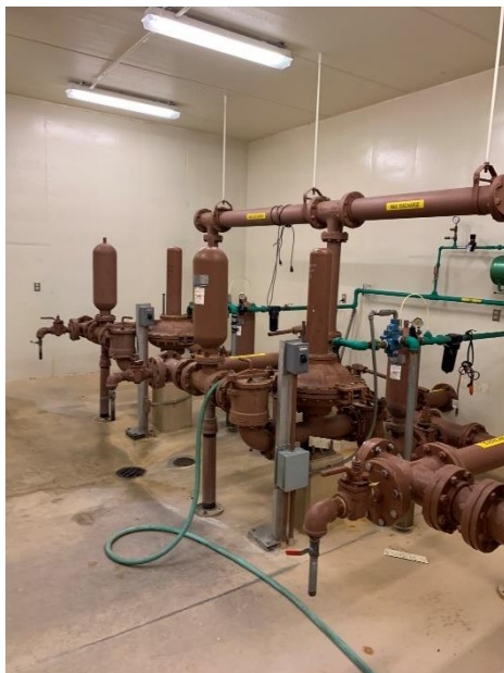
WAS Sludge Pumps & Compressors
