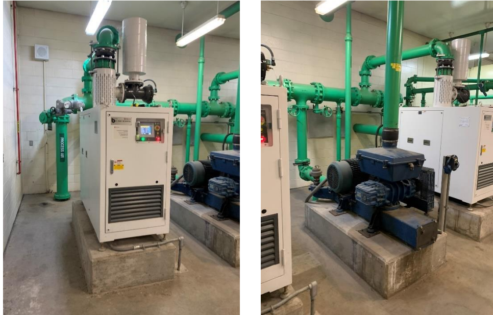
Turbo and Positive Displacement Blowers
