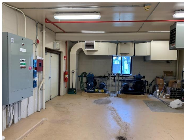
WAS Sludge Pumps & Compressors
